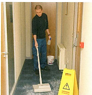
Milliken Capture powder is applied and agitated into the carpet and then thoroughly vacuumed.
